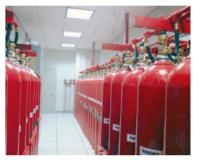
Gaseous fire suppression systems protecting machinery spaces, particularly in the case of smaller craft, may well incorporate scheduled extinguishing agents.
