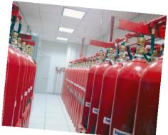
These clean fire protection agents preserve the desirable properties of Halon 1301 highly efficient, low toxicity, low chemical reactivity, electrical non-conductivity and high stability— and also have almost no impact on the environment. These properties, along with rapid detection and how quickly they work, make these agents excellent choices to protect marine vessels.
